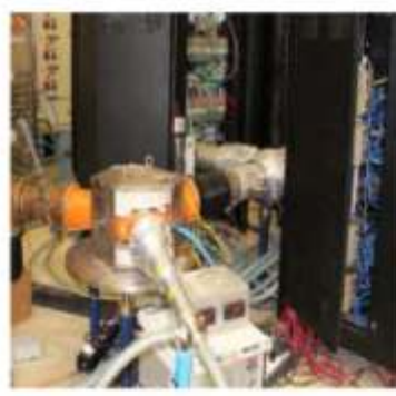
505.8 MHz RF Circulator for Indus-2
