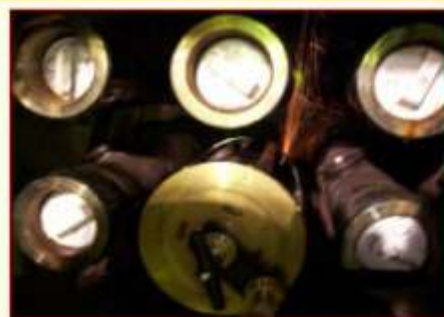
Laser cutting of bellow lips during en-masse coolant channel replacement (EMCCR) campaign in PHWR
